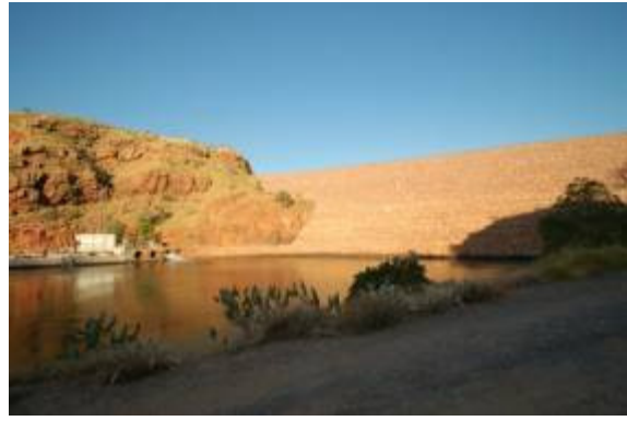
Figure 9: Lake Argyle dam wall and hydro-electric power station
